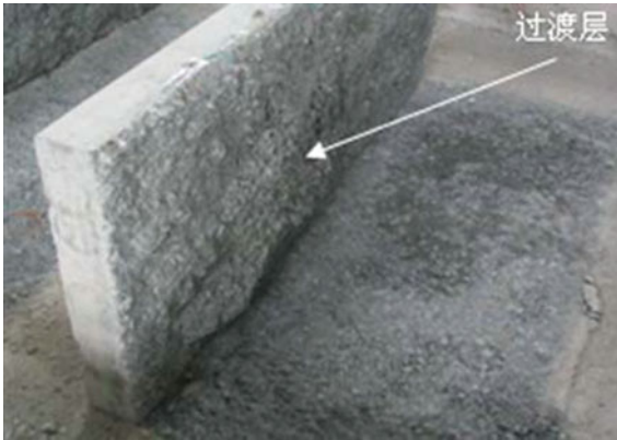
Fig. 1. Isolation layer of concrete pavement
